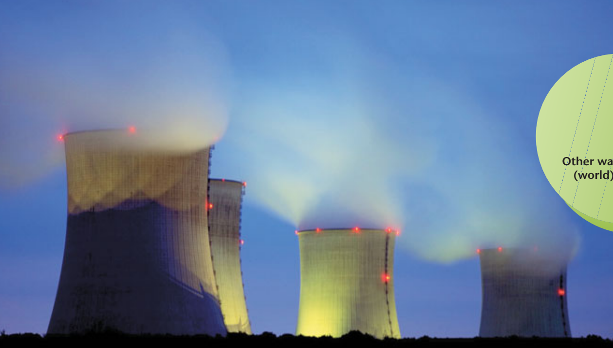
Figure 7 ► Water is a very important industrial resource. These nuclear power plant cooling towers release the steam produced from water used to cool a nuclear reactor.
