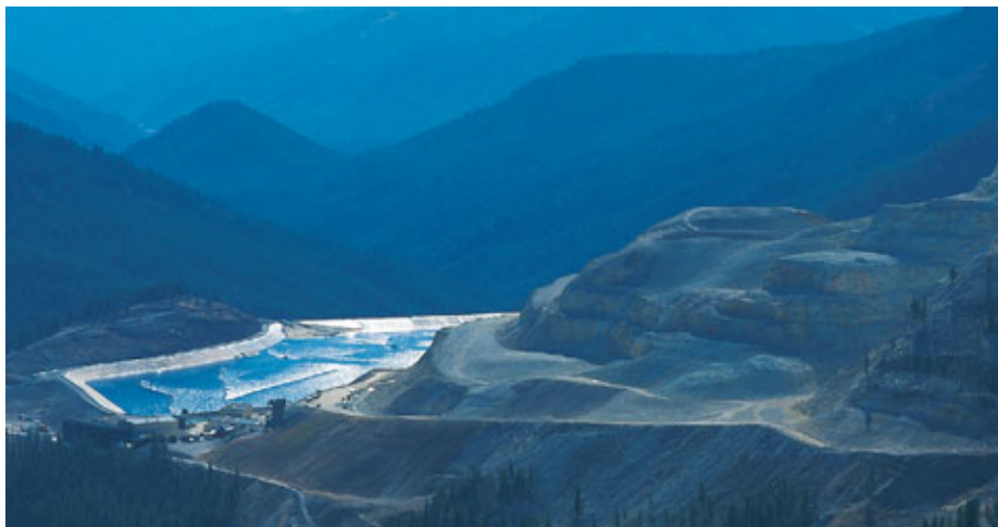
Figure 9 ► Cyanide heap leaching is being used to extract gold from ore at this open-pit mine in Idaho.
