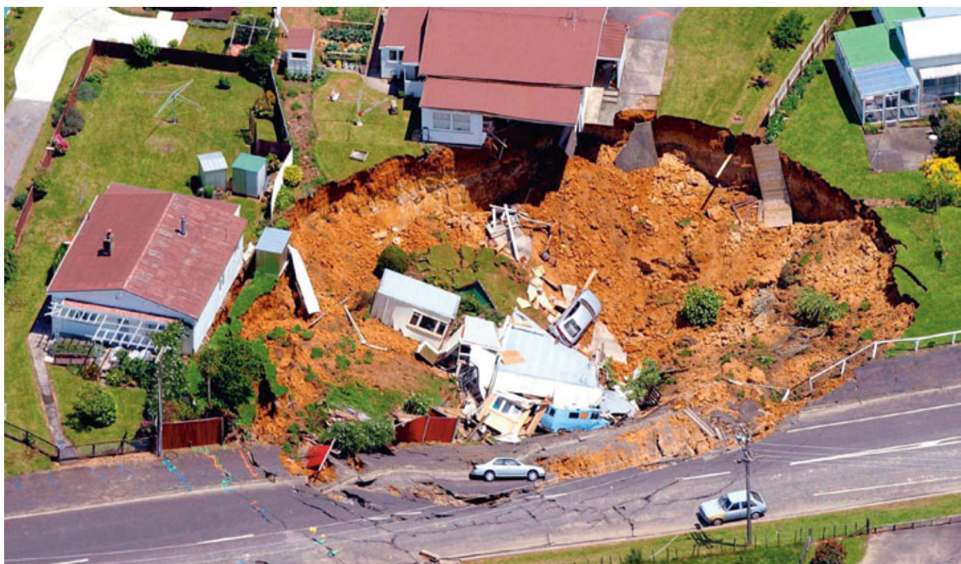
Figure 16 ► A hole created by the subsidence of a gold mine has swallowed this house in New Zealand.
