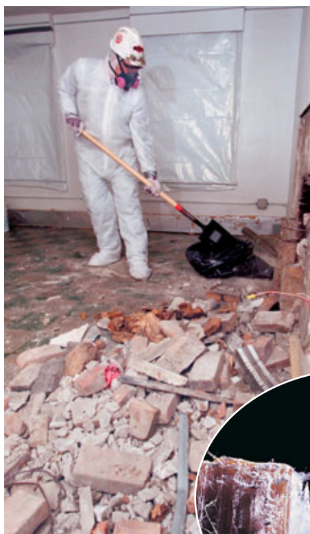
Figure 10 ► Asbestos (right) forms in long, thin fibers. The worker above is removing debris from a structure that was built with asbestos.
